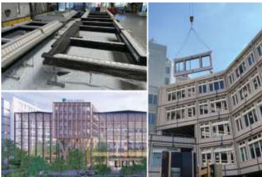
■ Façade elements for redevelopment of the ABN AMRO building use Duplicor biocomposites. Source | Duplicor
