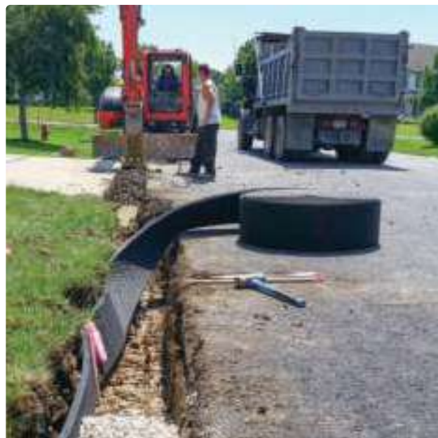
Applications for AWD’s drainage products include roadway edge drains as shown here.
