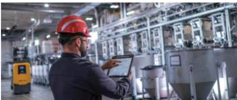
Above: Sun Chemical's mixing plant features high-speed mixers and the latest in digitalization and automation technology.
