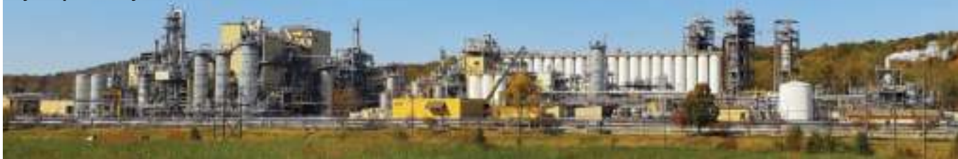
Syensqo's facility in Marietta, Ohio, US
