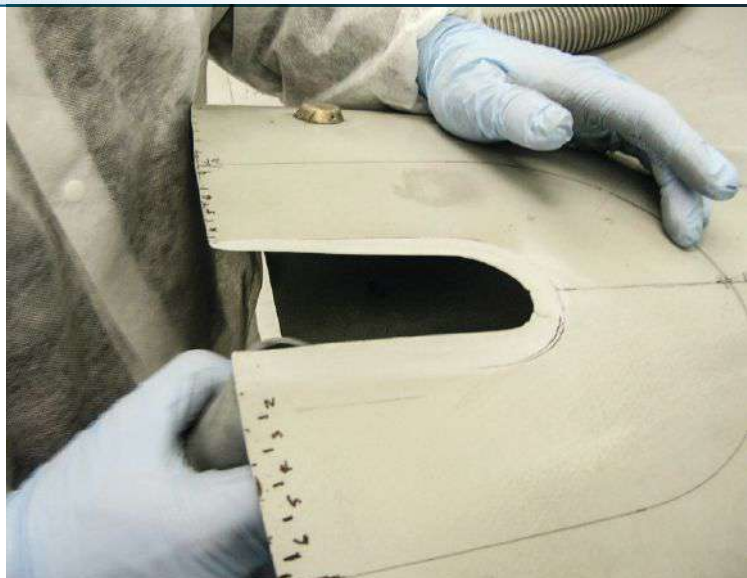
FIG. 1 Removal of damaged materials
