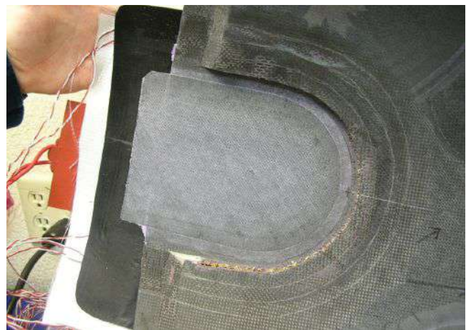
FIG. 4 Layup adhesives and repair plies
