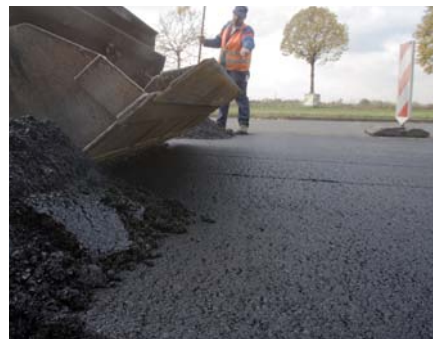
The use of VESTENAMER® improves the properties of the bitumen mixture and the processability of the asphalt.
